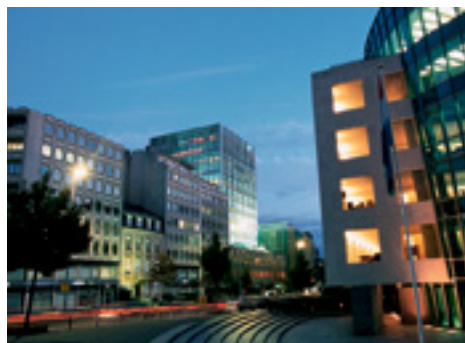
Completed new carrier structure in Europe
