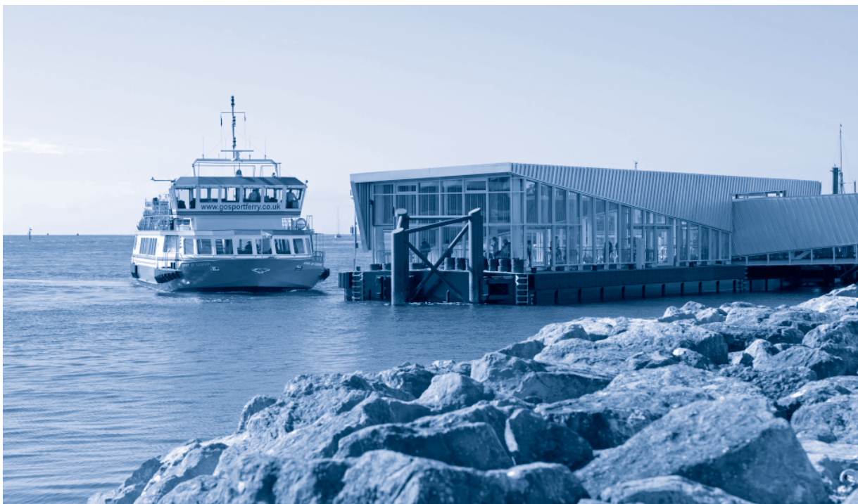
New pontoon at Gosport, installed in June 2011.
