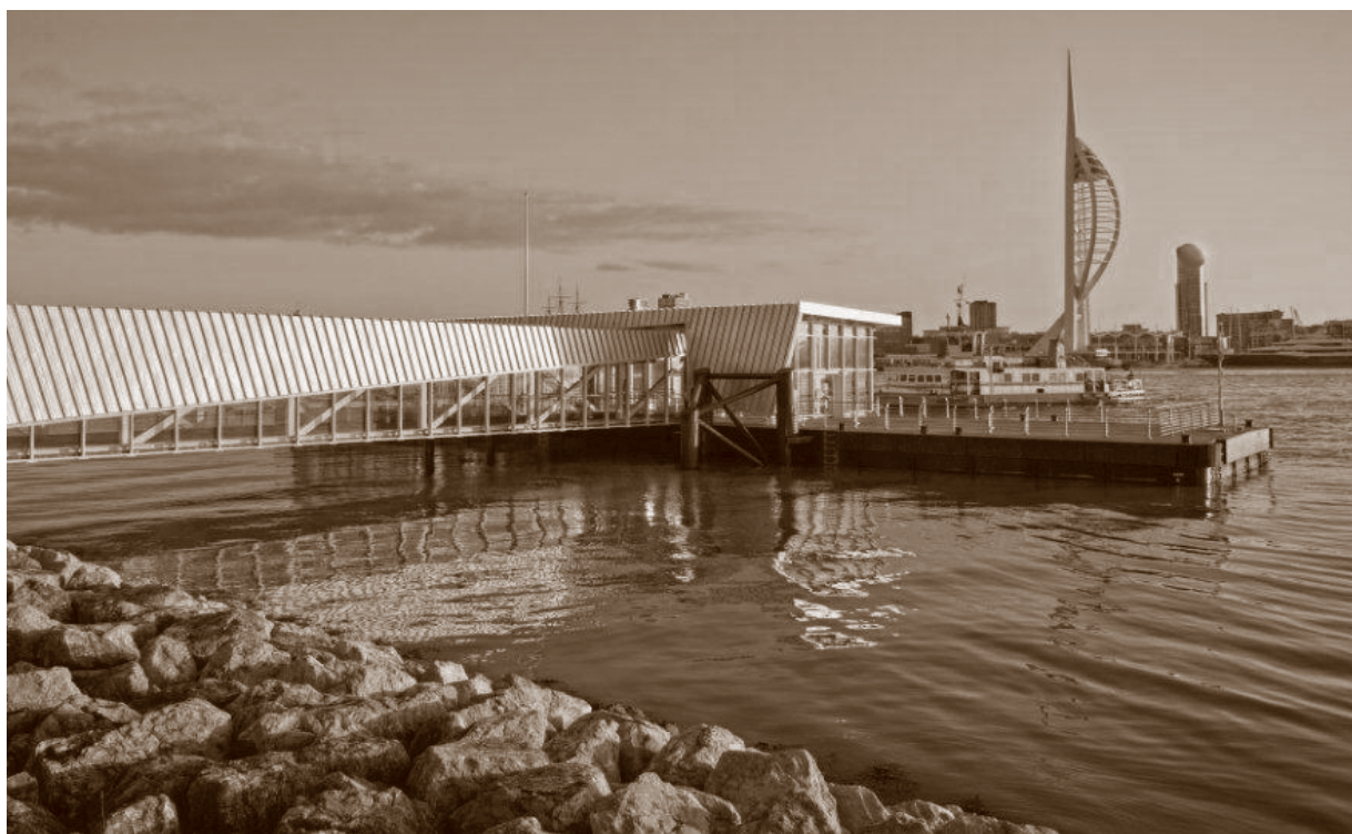
The new Gosport Pontoon installed June 2011.
