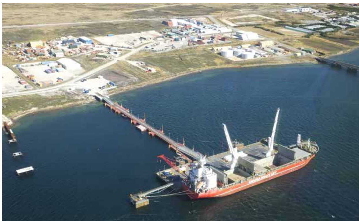
Temporary floating dock, this photo has been reproduced with the permission of Stephen Luxton
