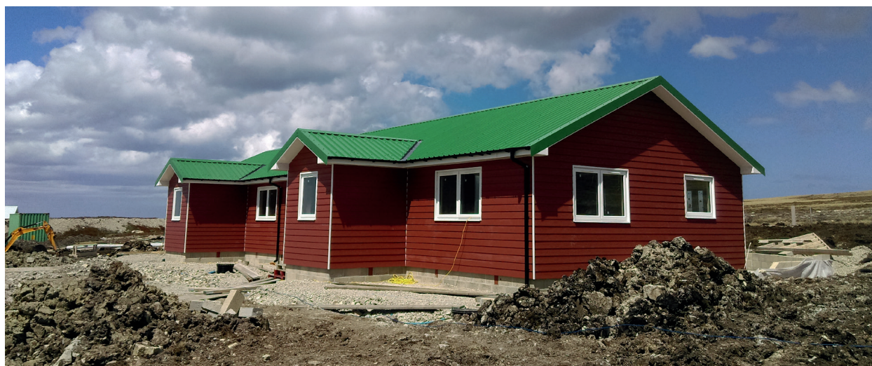
A newly constructed house, built for the Falkland Islands Government
