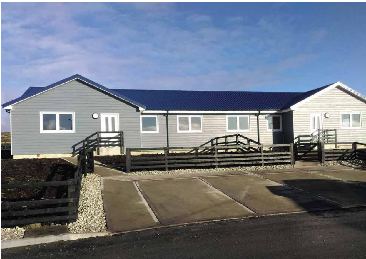
Housing built by Falklands Building Services
