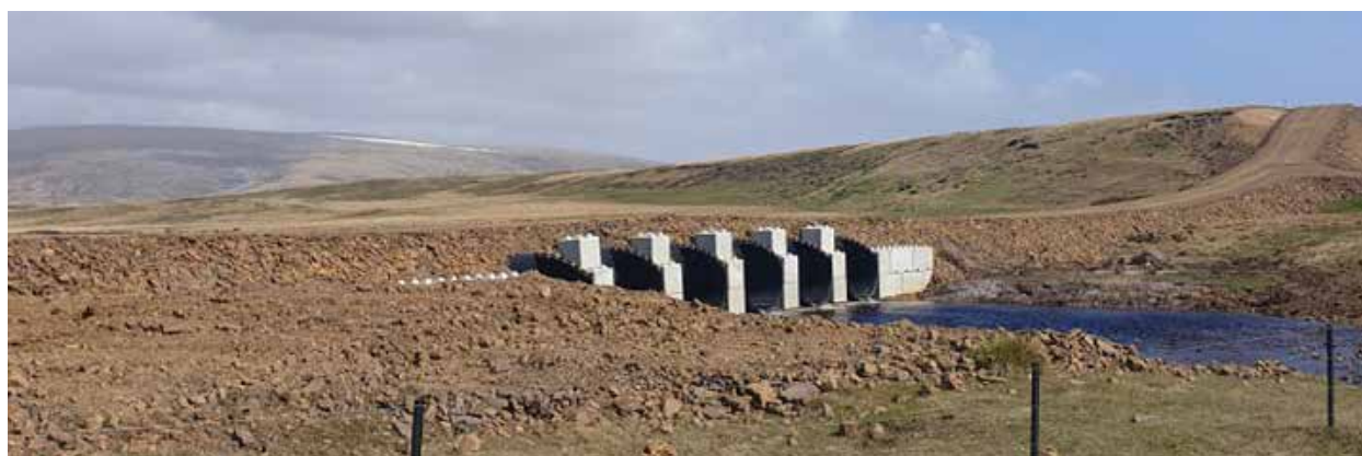
Newly constructed culverts built for the Falklands Islands Government
