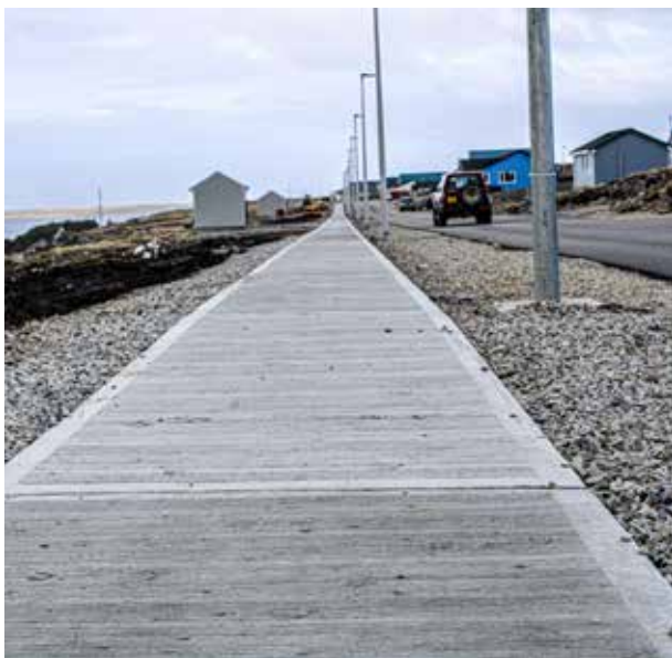
FIC constructing a path
