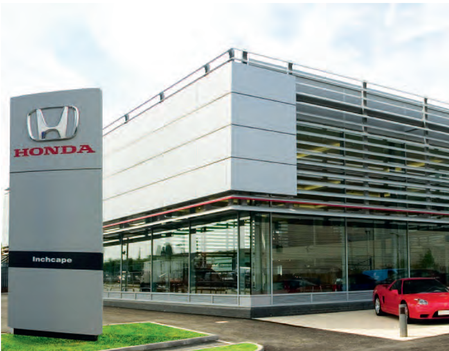
By recycling rainwater, using ground source heating pumps and solar power to heat water, Incape Honda in Romford, UK uses around 30% less energy than a standard car showroom.
