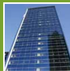
380 LATROBE STREET MELBOURNE, VIC
