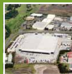
NXQ DISTRIBUTION CENTRE PINKENBA, QLD
