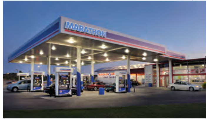
This outlet in Muskegon, Mich., is owned by Marathon Flint Oil Co., which has been a Marathon jobber for 65 years.
