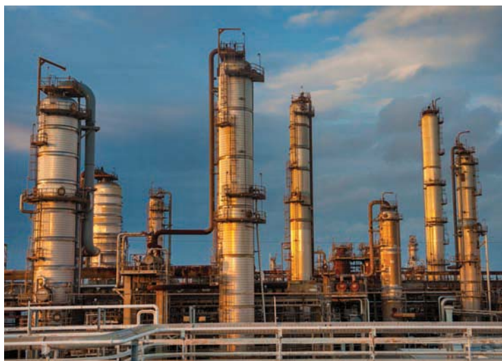
Above, aromatic recovery unit at the Galveston Bay refinery's West Plant
