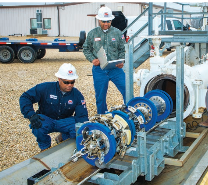
Technicians prepare an in-line inspection tool to evaluate a pipeline.
