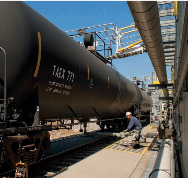
Railcars at MPC's Canton, Ohio, terminal
