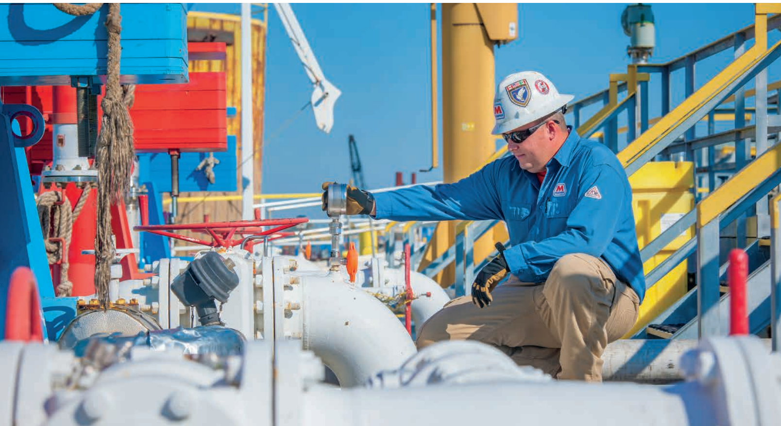
Loading dock at Wood River, Ill.
