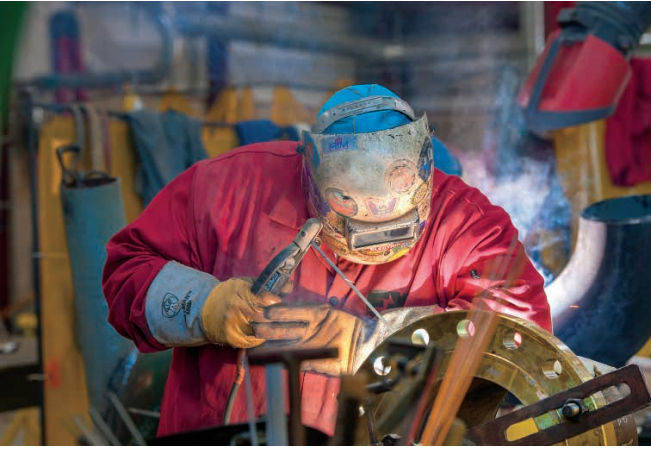
Maintenance work at our Robinson, Ill., refinery
