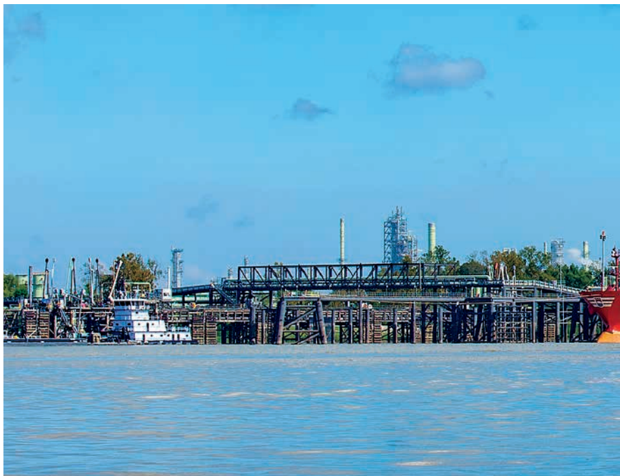
Export dock on the Mississippi River at MPC's refinery in Garyville, La.
