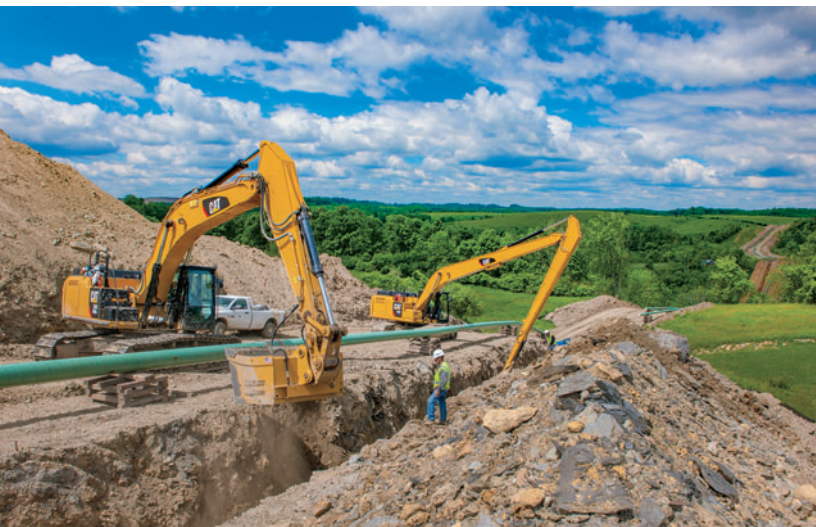
Laying pipe for MPLX's Cornerstone Pipeline
