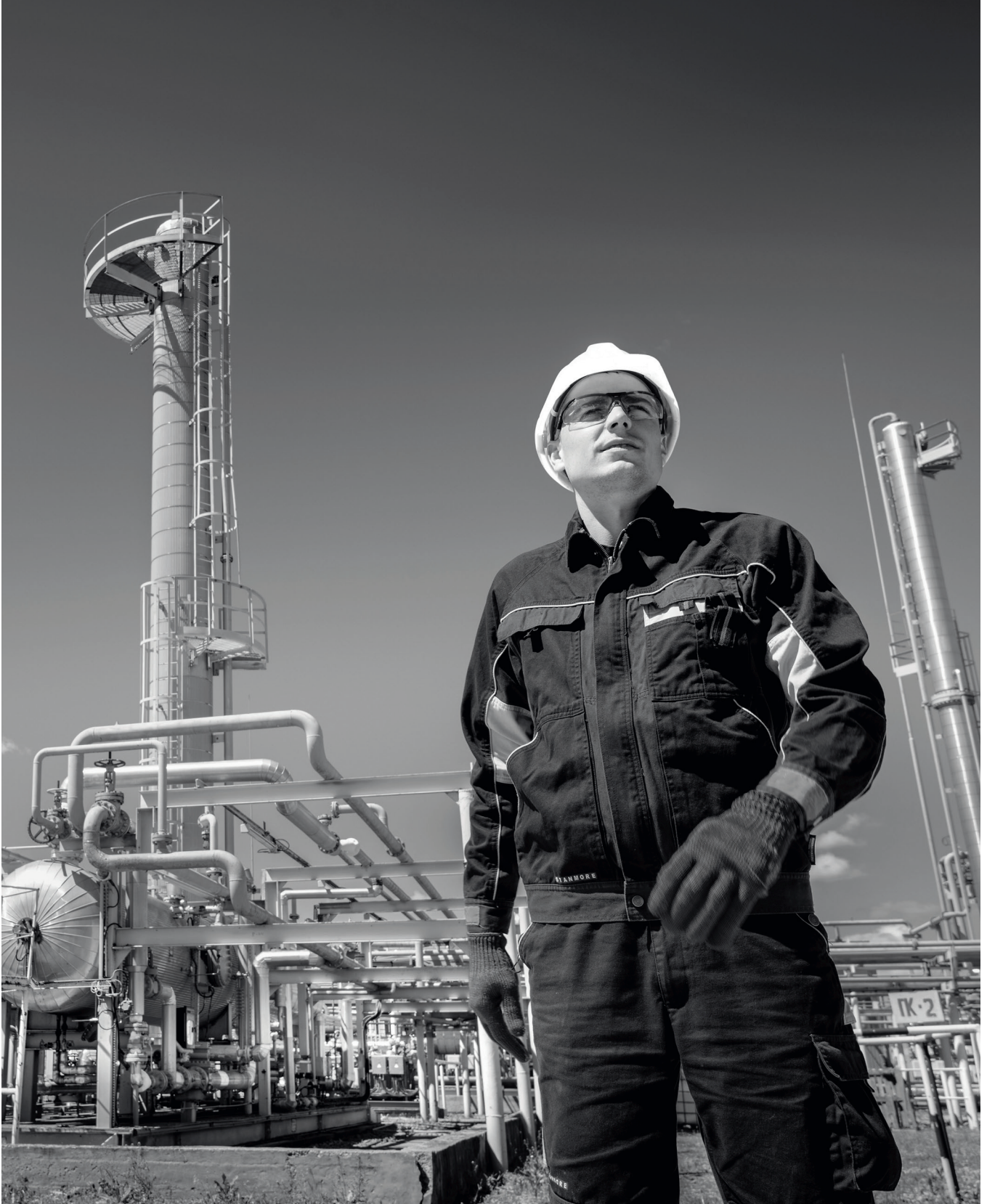
LPG plant at the Sakalova Balka production facility in Ukraine.
