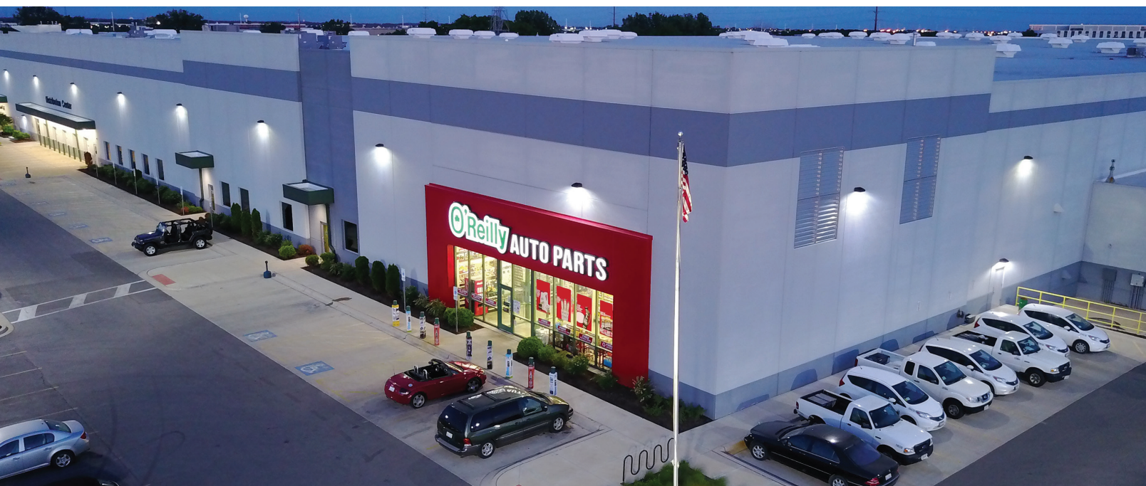
Naperville, IL, Distribution Center.
