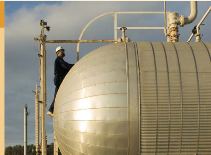
A plant operator inspects LP storage tanks in Waskom, Texas to insure safety and efficiency.
