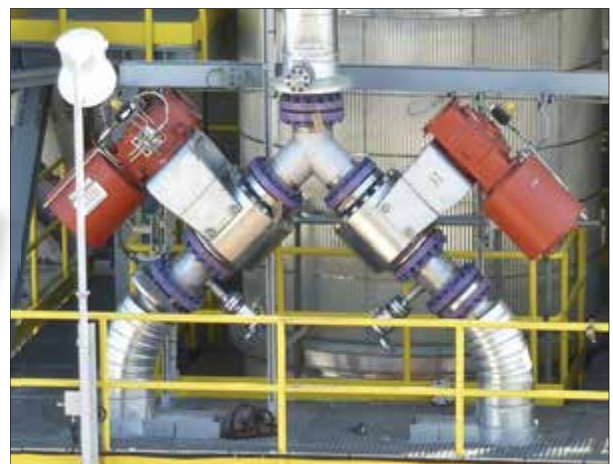
Velan 10" Class 150 Securaseal™ severe service ball valves installed in a nickel mining facility.
