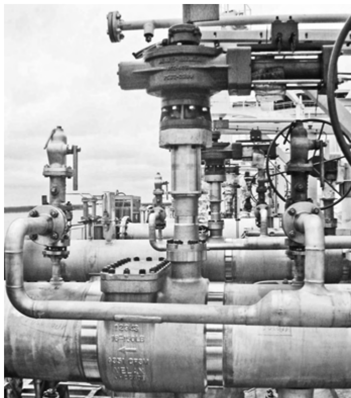
16" Velan Velflex cryogenic butterfly valve on an LNG Carrier.
