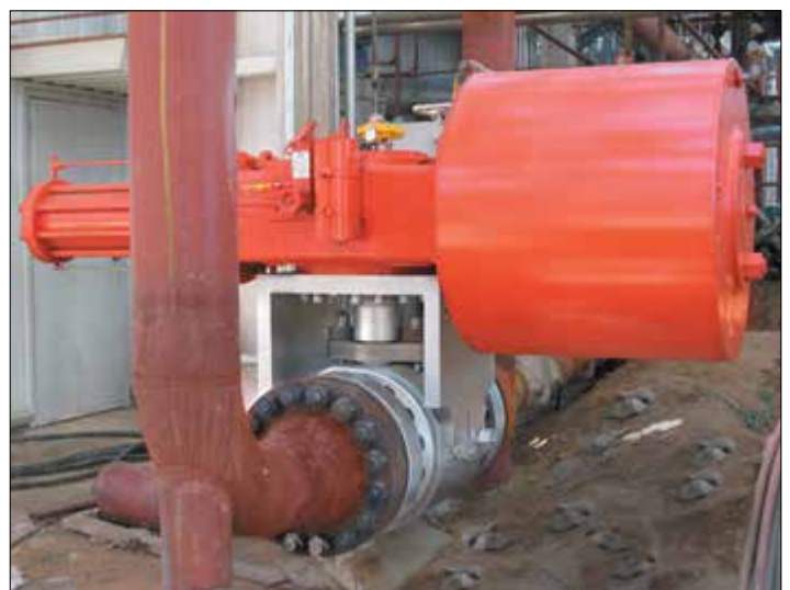
A Velan pneumatically operated metal-seated ball valve used for isolation in a hydrocracking unit in Asia.
