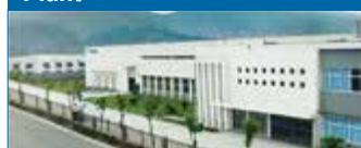
Suzhou, China Velan Valve (Suzhou) Co., Ltd.
