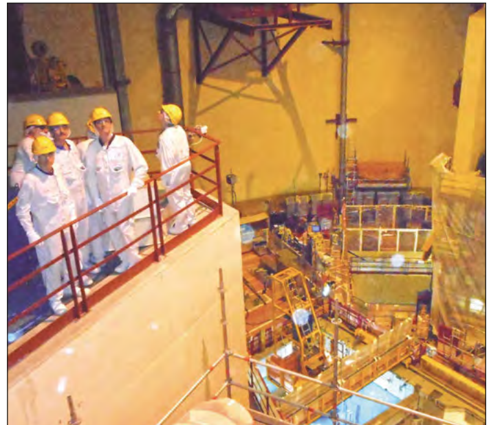
Velan executives visit a nuclear plant in France where there is a large installation of Velan valves.
