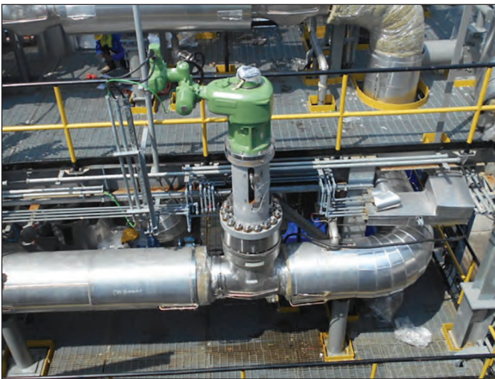
Velan 16" Class 2500 forged gate valves for high pressure and high temperature Hydrogen service installed on an AXENS-HYVAHL process at IRPC Rayong facility in Thailand.
