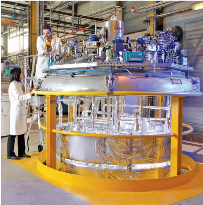
Velan SAS manufactured these cryogenic bellows seal globe control valves for liquid helium application installed in a nuclear fusion reactor in Japan. Photo credit: P.AvavianCEA.
