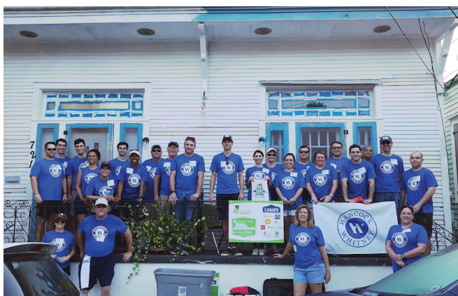
Rebuilding homes and lives. Local associates joined Rebuilding Together's Build A Healthy Neighborhood national project to help repair homes in New Orleans' historic St. Roch area.
