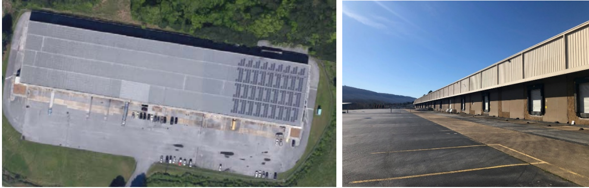
Photo: PUREgraphite's new home in Chattanooga Tennessee USA.
