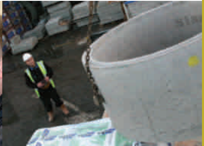
Loading pipe sections at Keyline, Hull
