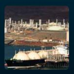
At the onshore *Karratha Gas Plant*, raw gas is processed and separated into pipeline gas, LPG, LNG and condensate.
