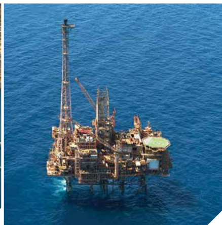
The Greater Western Flank Phase 1 Project is a subsea tieback to the Goodwyn A platform.
