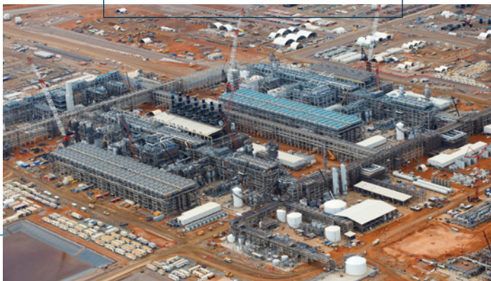
All Wheatstone Project Train 1 and Train 2 modules are set on their foundations.
