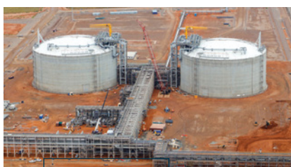
LNG storage tanks being completed.
