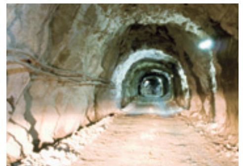
Below: Tunnel at the San José operation.
