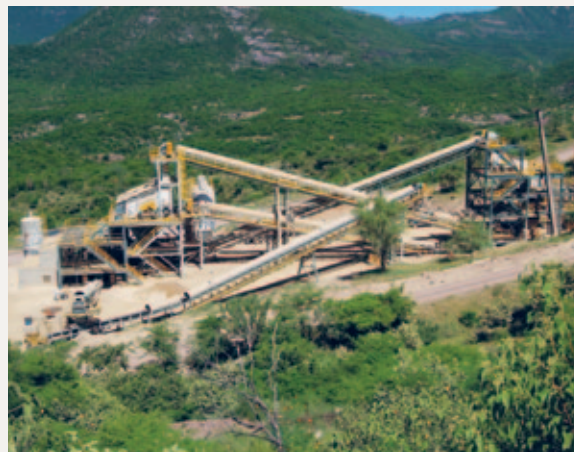
View of the plant at Moris
