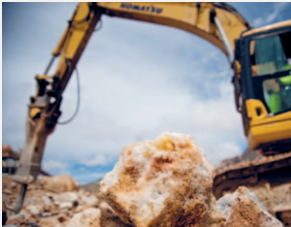
Work in progress at Pallancata
