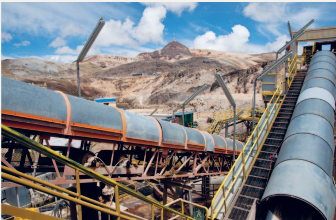
View of the Selene plant
