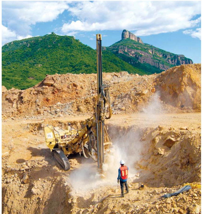
A drill rig in operation
