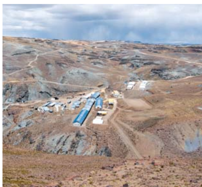
View of the Inmaculada Advanced Project
