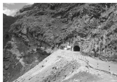
Ramp at Pallancata
