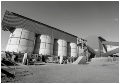
San Jose plant
