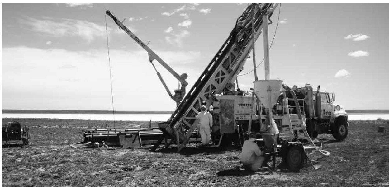
Drill rig in Argentina
