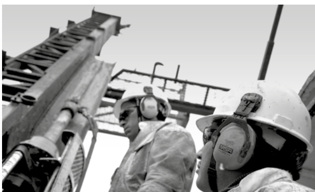
Drill rig at Azuca
