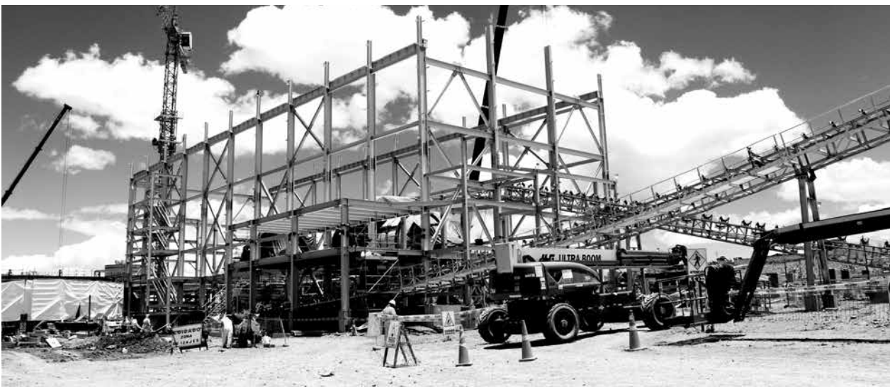
Inmaculada plant construction
