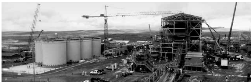
Inmaculada plant construction
