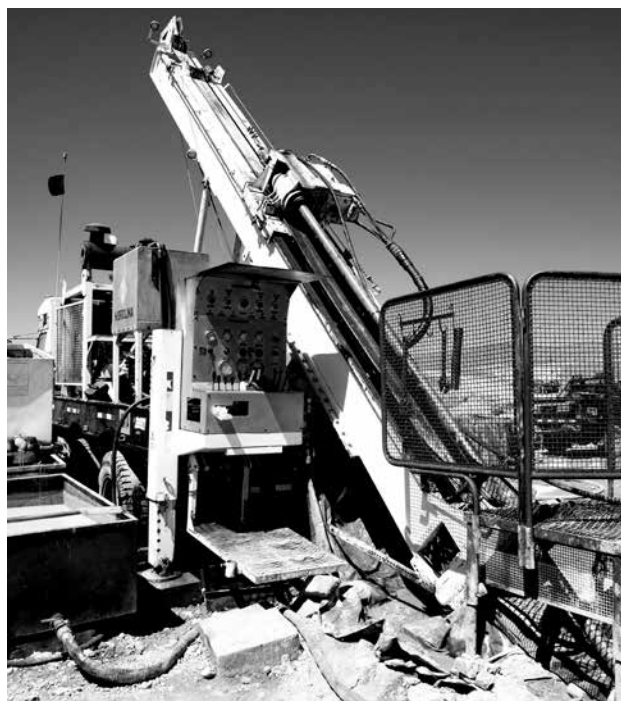
Drill rig at Pallancata
