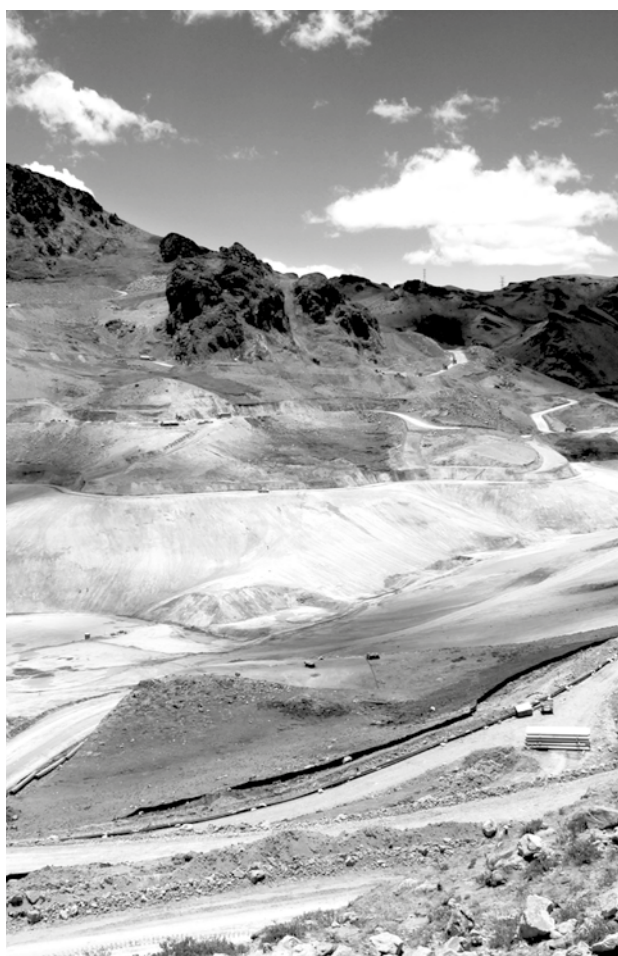
Tailings dam preparation
