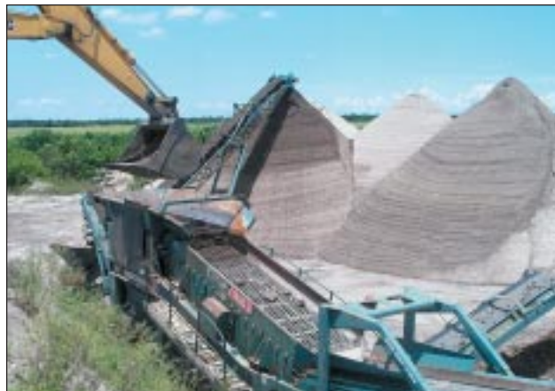
Screening material for fill dirt
