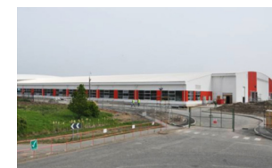
Sunderland automotive battery plant
