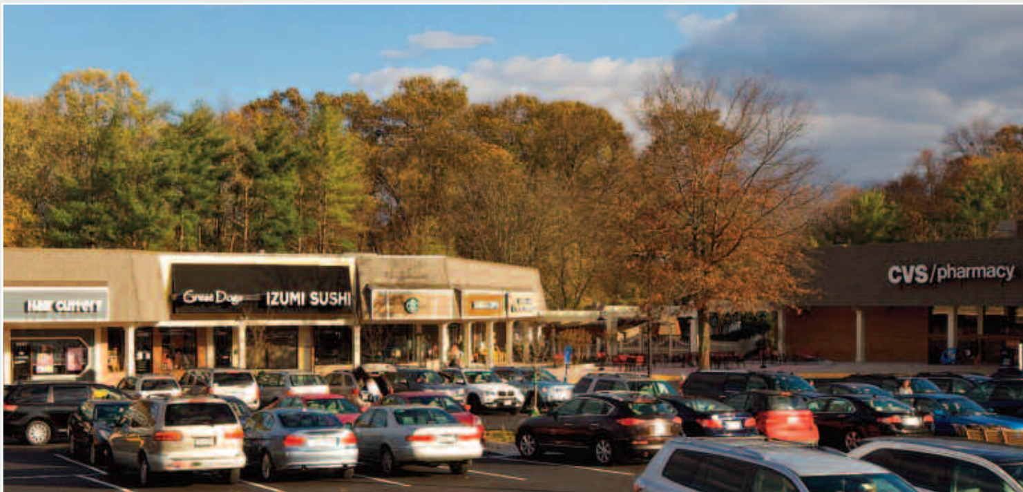
Great Falls Center (recently renovated), Great Falls, VA
