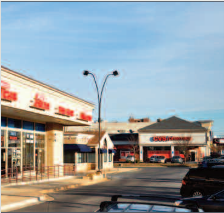
Development site, Twinbrook Metro, Rockville, MD
