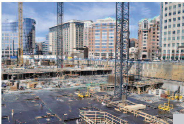
750 N. Glebe Road, Arlington, VA (construction in progress)
