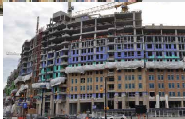
CONSTRUCTION IN PROGRESS
