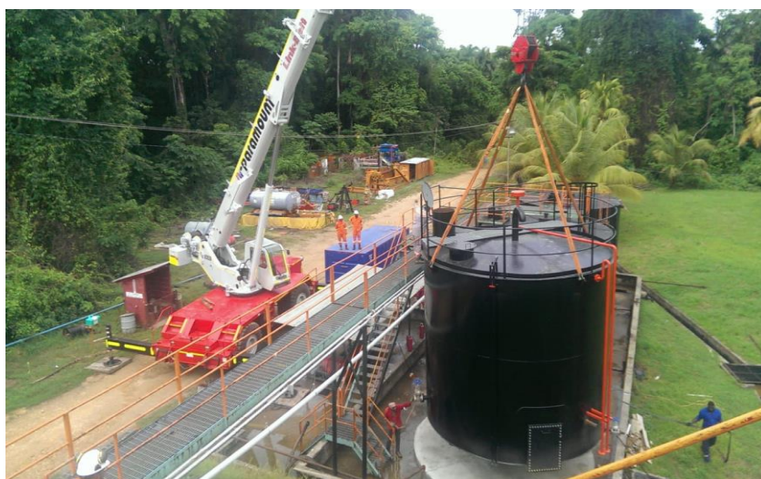
Installation of a new storage tank
