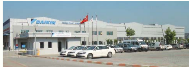
A Group company in Turkey has begun manufacturing air-conditioner products designed to match local needs.
