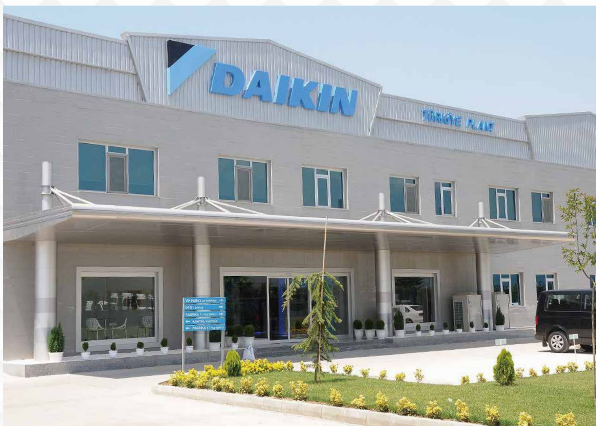
Daikin's plant in Turkey goes into full-scale operation.
