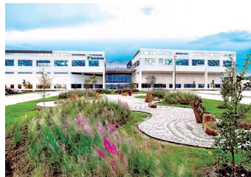
Daikin Texas Technology Park where production, development, logistics, sales, marketing and indirect departments work together to create a constant flow of innovation.
