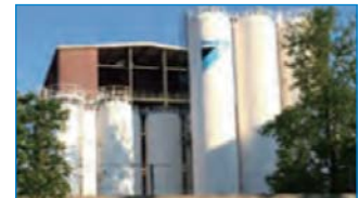
Refrigerant reclamation and destruction facility in Germany, part of a scheme for the recovery, reclamation and destruction of refrigerant
