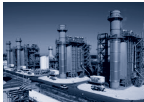
Tampa Electric recently completed upgrading Polk Power Station, expanding capacity by about 460 MW.
