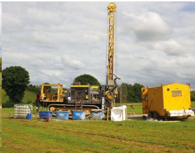
Drilling Clay Lake.
