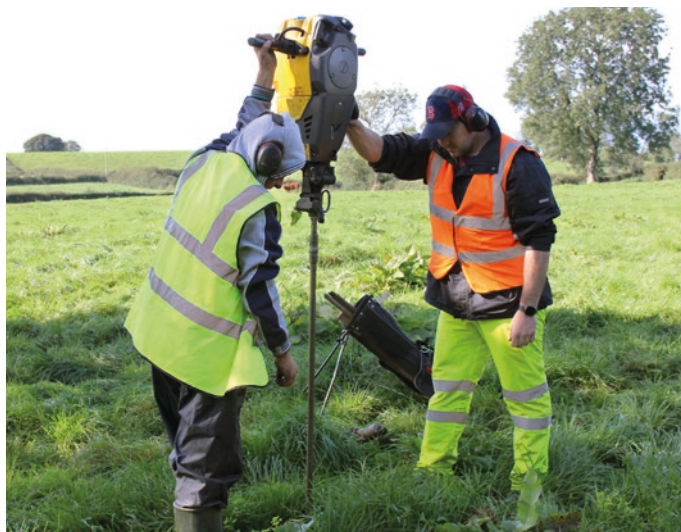
Deep overburden sampling.
