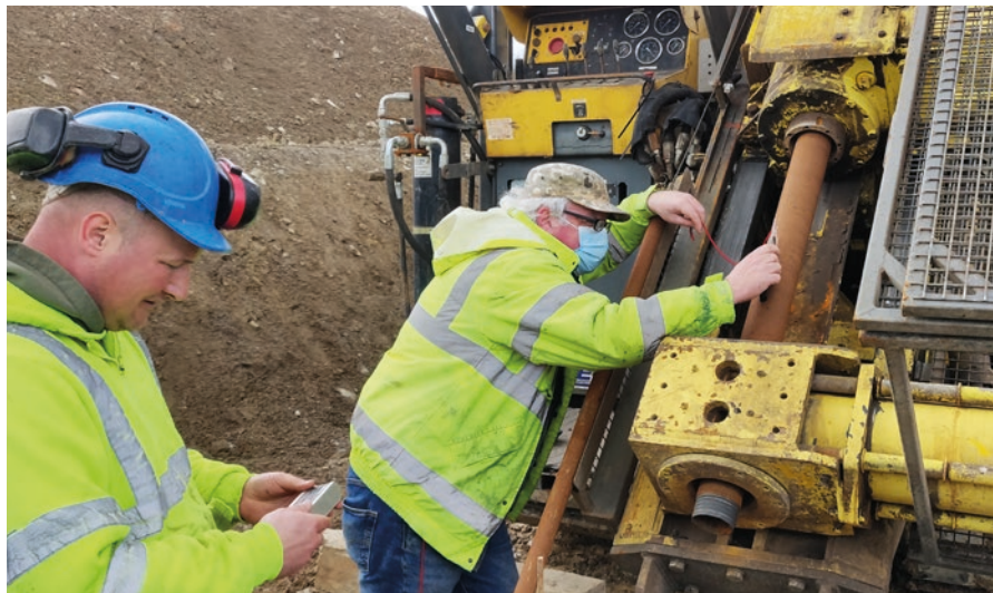
Setting up drill rig, Clontibret.
