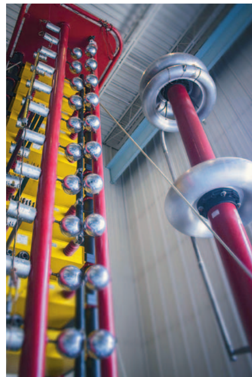
Advanced testing is performed inside Doble's High Voltage Laboratory including endurance testing, research on dielectric behavior, failure analysis and partial discharge detection.
