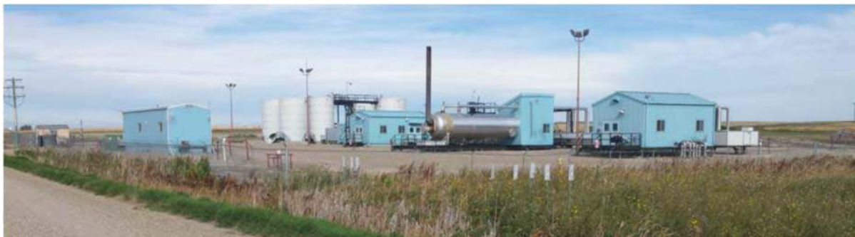
Representative Asset Oilfield Production Facilities (Little Bow Oilfield Battery)
