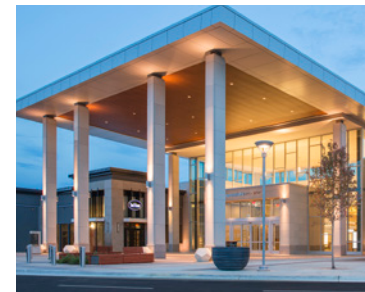
SPRINGFIELD TOWN CENTER Springfield, VA Ownership Interest 100% Acquired 2015 Square Feet 1,374,000
