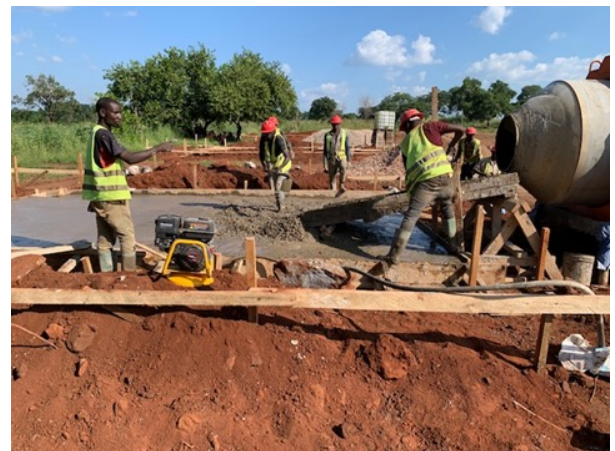
Concreting Works on site
