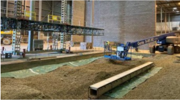
Construction of Cathode Wet Mixing Room
