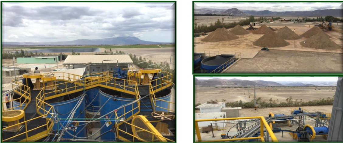
Figures 1 to 3: Vista Gold Plant – Leach Tanks for gold recovery (left), Crushed ore stockpiles ready for grinding and processing (upper right), and ball mill grinding circuit and conveyor feed to leach tanks (lower right)
